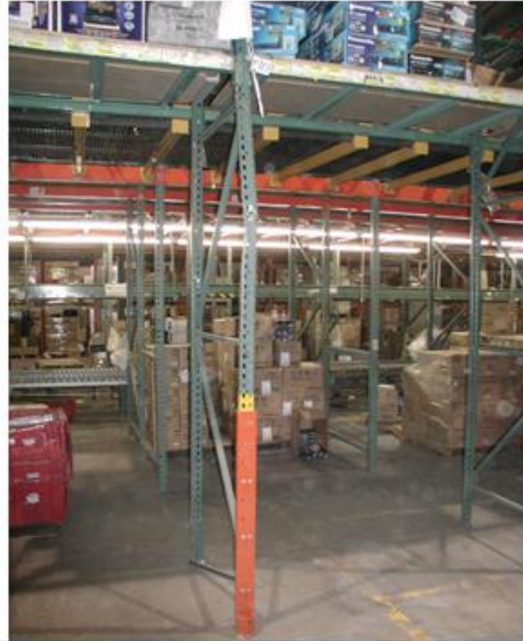
Damaged column with home grow repair
