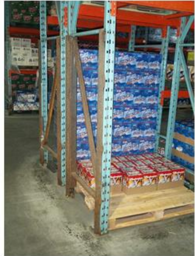
Unsafe Field Bracing Repair
