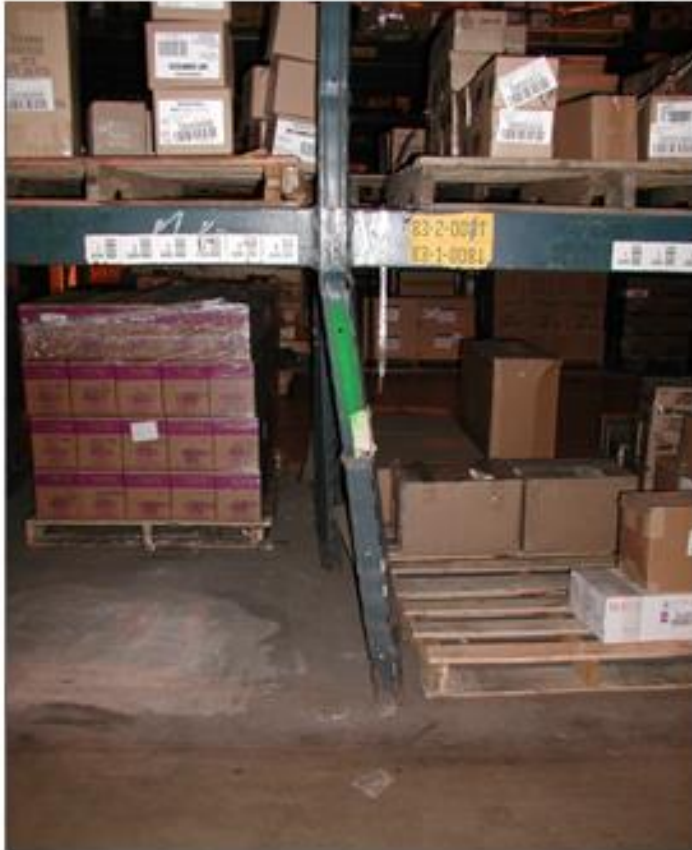
Damaged Upright Column
