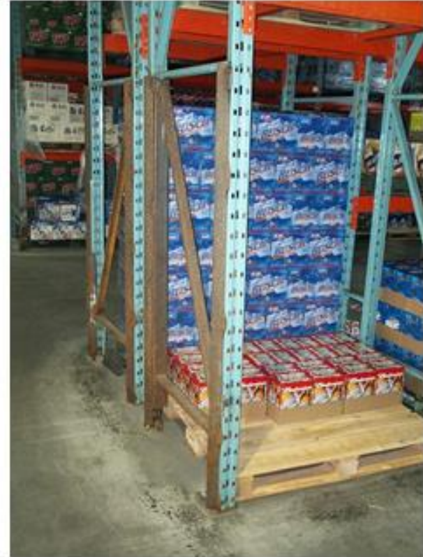
Unsafe Field Bracing Repair
