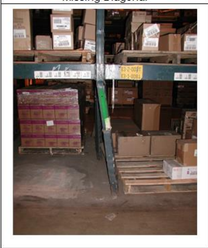
Damaged Upright Column
