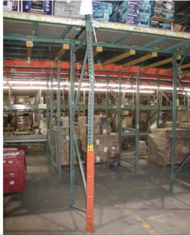
Damaged column with home grow repair
